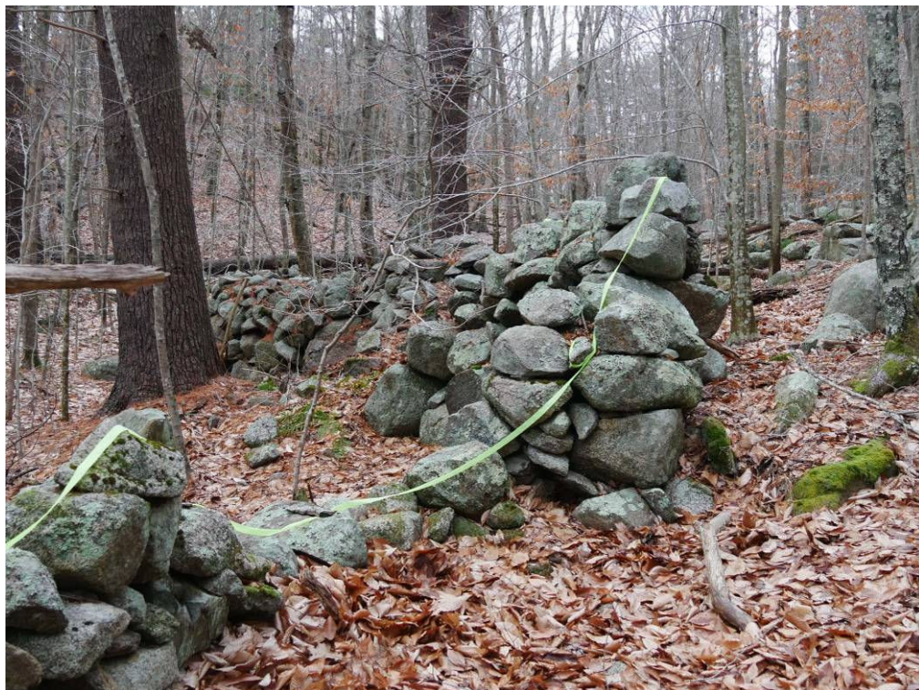
Finished end of wide wall & low wall section
