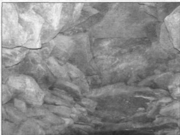
Figure 15. Inside photo showing the corbelled domed roof of a chamber in Thompson, Connecticut.
