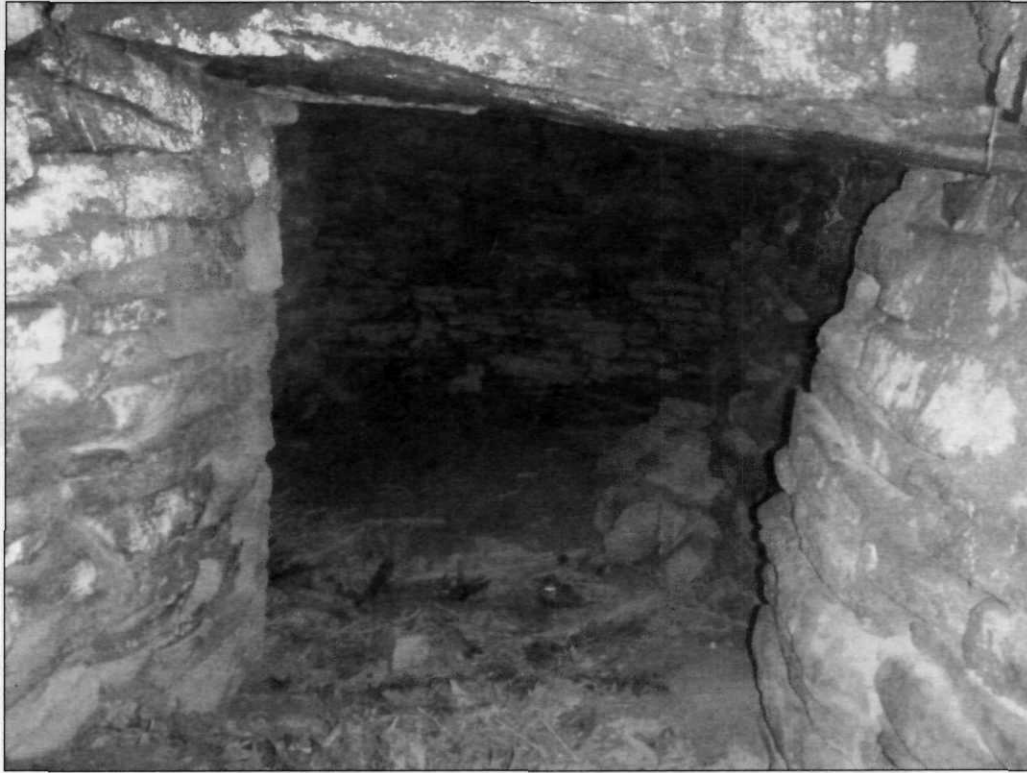
18B. Above, interior Room – Straight vertical walls, square corner, flat faced stonework.
