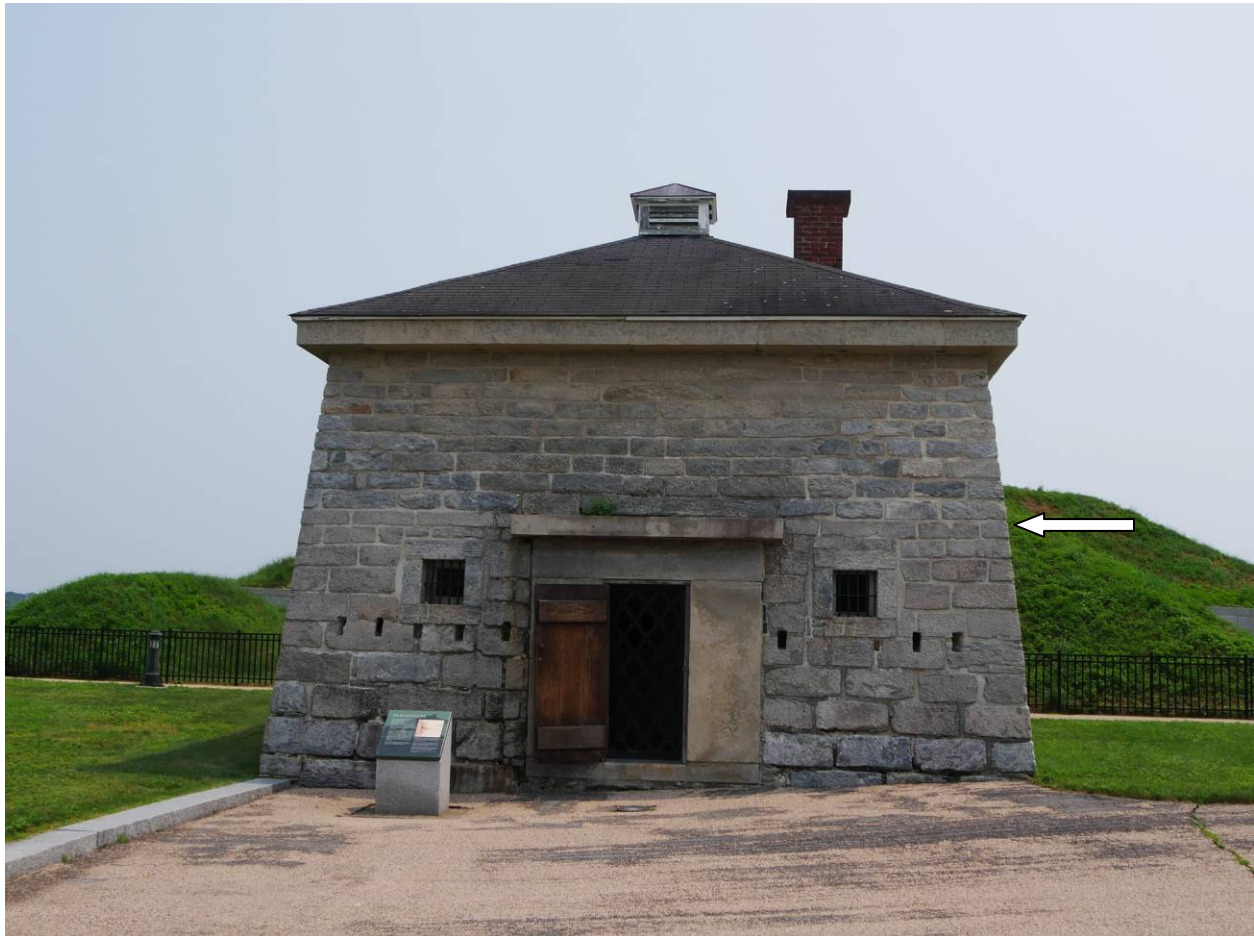
Figure 1 – West side of block house with entrance. The top layer of the original 1794 block house is indicated by the arrow. It has the same height as the entrance.
