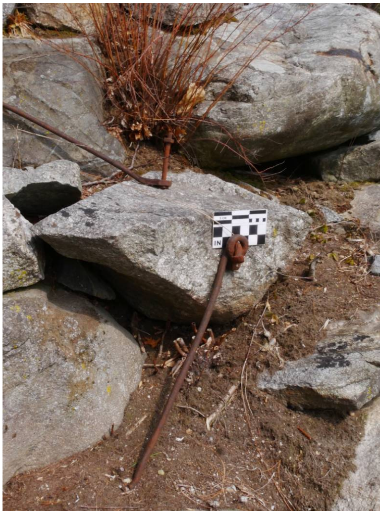
Figure 6 – Metal rods attached to the eyebolts use to secure the “summer house” a small building on the mound in the 1930s.
