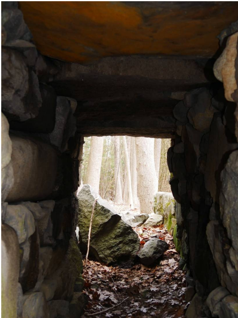
Figure 12a – Interior of the tunnel
