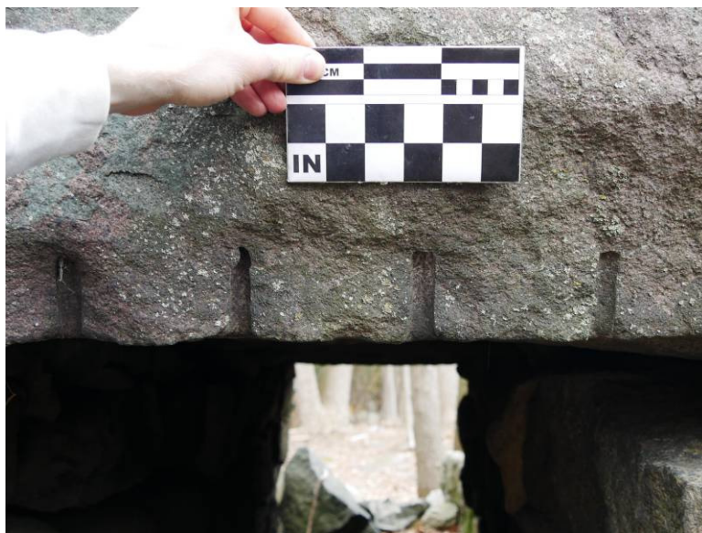
Figure 13 – Plug & feather half round drill marks.
