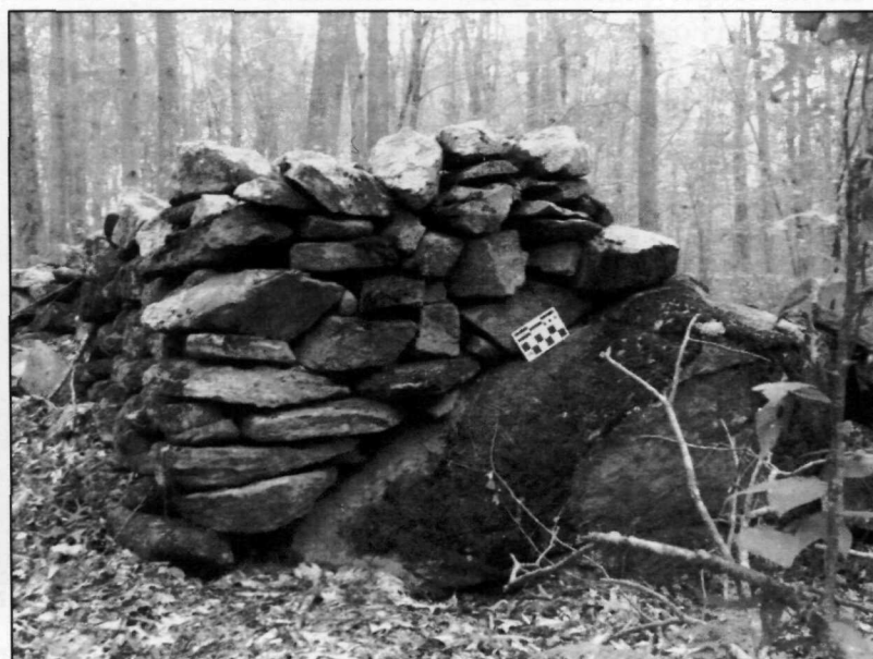
Figure 3. The vertical wall of this cairn exhibits Euro-American style construction in which one stone covers the joint of the two stones below it (#1698, West Side – Jonathan Foster Farm).
