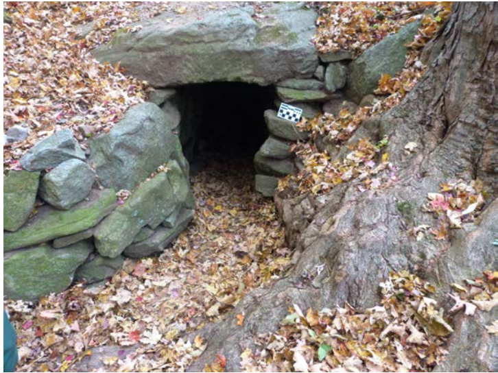
Upton Chamber: OSL samples were taken from the builders trench behind the left hand entrance wall.
