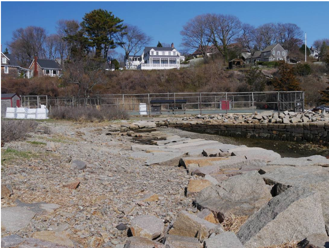
A tennis court now covers the bottom of quarry #1. The ledge face of the quarry is obscured by vegetation.
