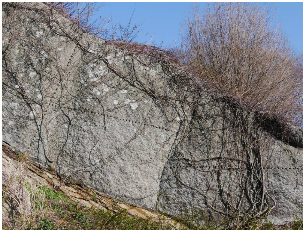
Vertical and horizontal lines of closely spaced drill holes (on eastern ledge)
