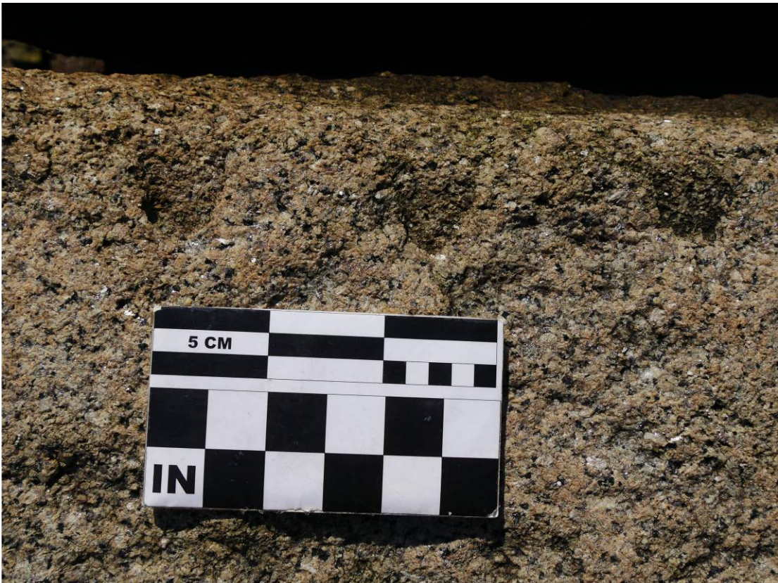
Examples of quarry tool marks made by the flat wedge method. Holes are worn from storms.
