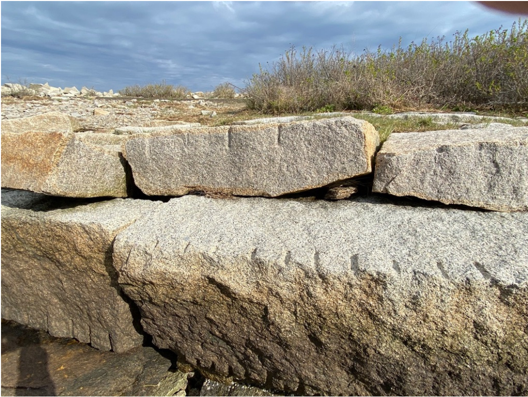
Half round quarry holes from the plug and feather method
