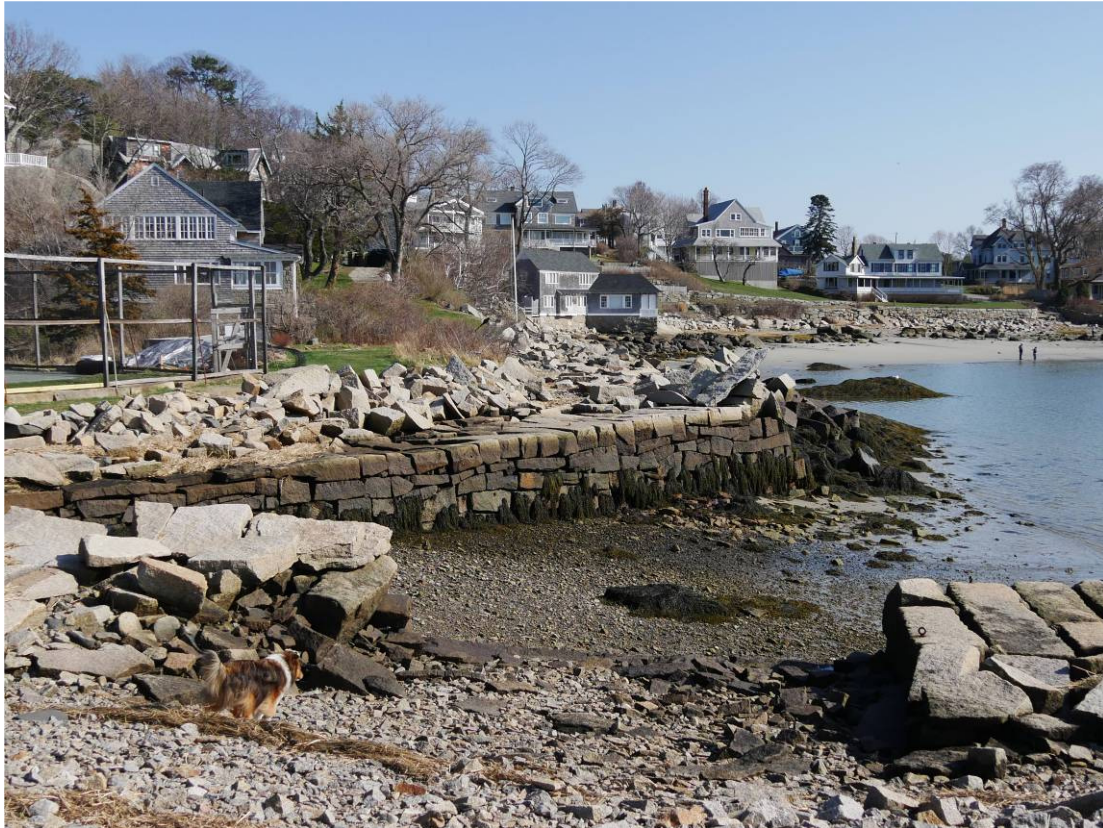
The first section of the wharf which parallels the shoreline.
