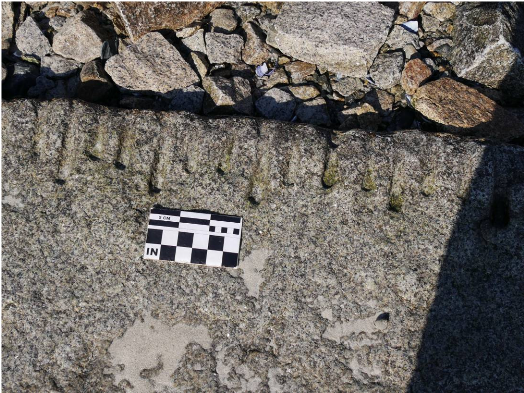
Closely spaced half round holes with alternating depths, part of an effort to split some difficult to quarry granite
