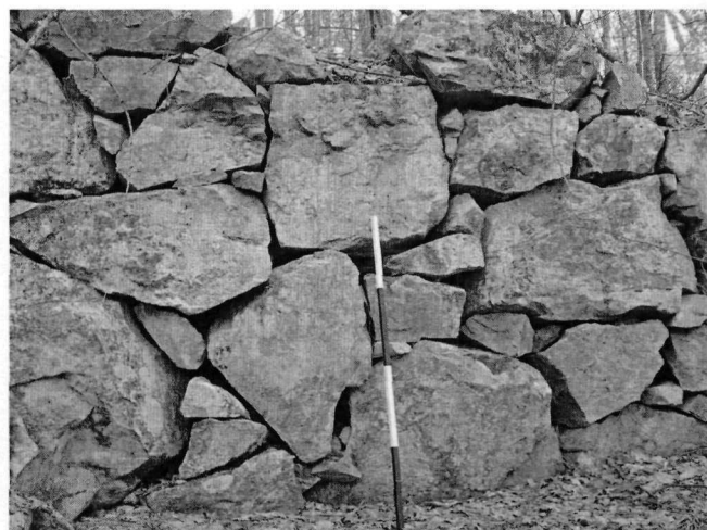
Figure 10. Pingree Barn, Georgetown, MA – extra large blocks and large blocks of stone were the primary stones, some of the extra large blocks had blast hole marks. There were no small quarry hole marks on any of the stone.
