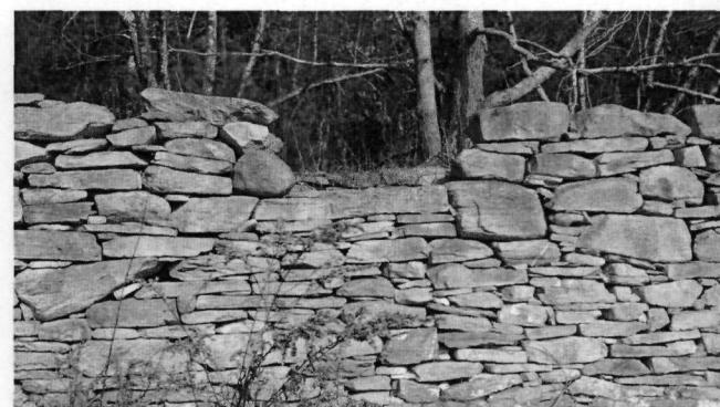
Figure 11. Barn foundation at Farm Site, Thompson, CT – Slabs of stone (larger than used in the house foundations) with sharp edges. Lengths and thickness vary.
