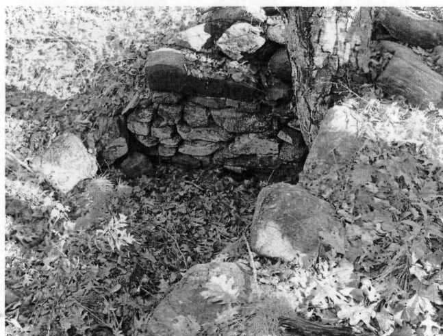
Figure 5. House foundation, Crowd Site, Sturbridge, MA - Rectangular blocks with rounded edges.
