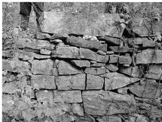
Figure 4. House foundation, Hampstead Forest, Hampstead, NH - Rectangular blocks with sharp edges.
