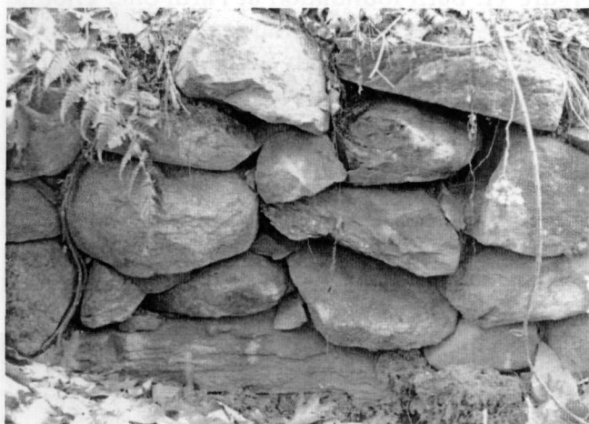
Figure 3. House Foundation, Bugsmouth Hill, South Hampton, NH – Cobble stones with semi-flat faces.
