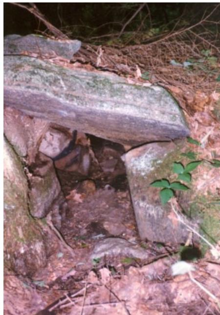
Fig. 10 - A typical stone culvert under a road (Governor's Island, Hampstead, NH)
