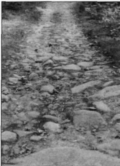
Fig. 15 – Stone used to repair road in Canton, Maine.
