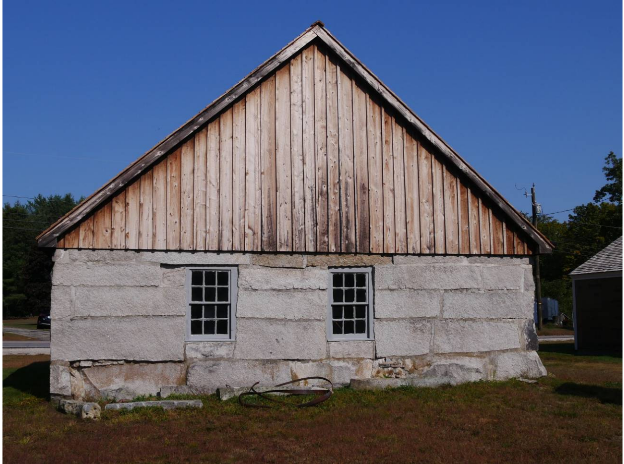
Rear wall of shop. Poor quality stone slabs were used for the layer at ground level. Some bars with orange stains were used as lintels near the roof line. The second story was wood on this end unlike the front of the shop where stone was used.
