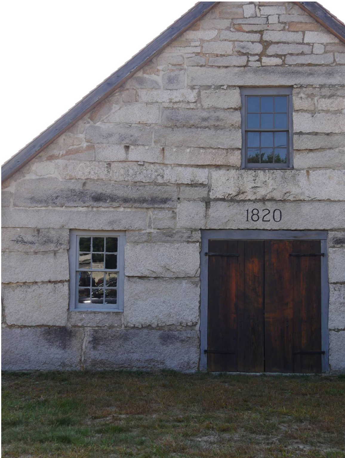
Front of Blacksmith Shop. The largest stone blocks and bars were used to construct the first story of the building. The second story of building shows a gradually decrease in the sizes of the stone with height. The notable exception being the lintel stone over the window.
