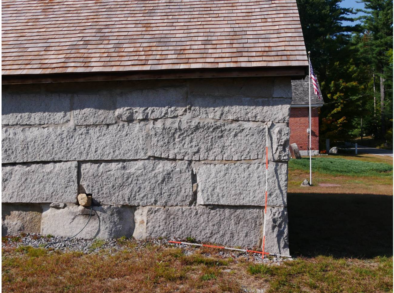
Left side wall of shop. Photo scales are marked in one foot intervals. The stone is of a uniform color and texture suggesting it came from the same source, either a large glacial erratic or surface ledge quarry.
