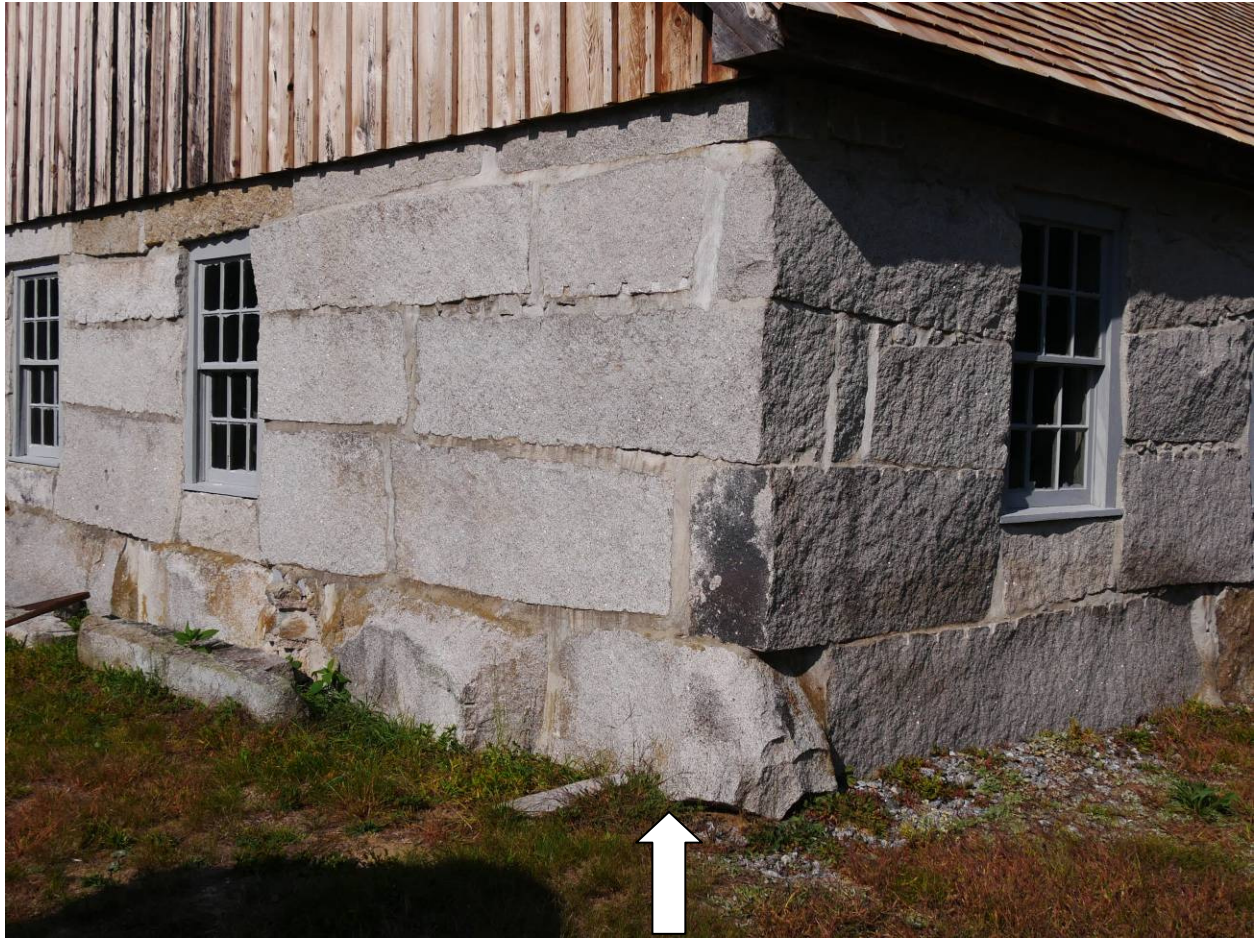
Angled view of rear shop wall. Arrow indicates a block with some non-flat surfaces utilized in the least conspicuous place.
