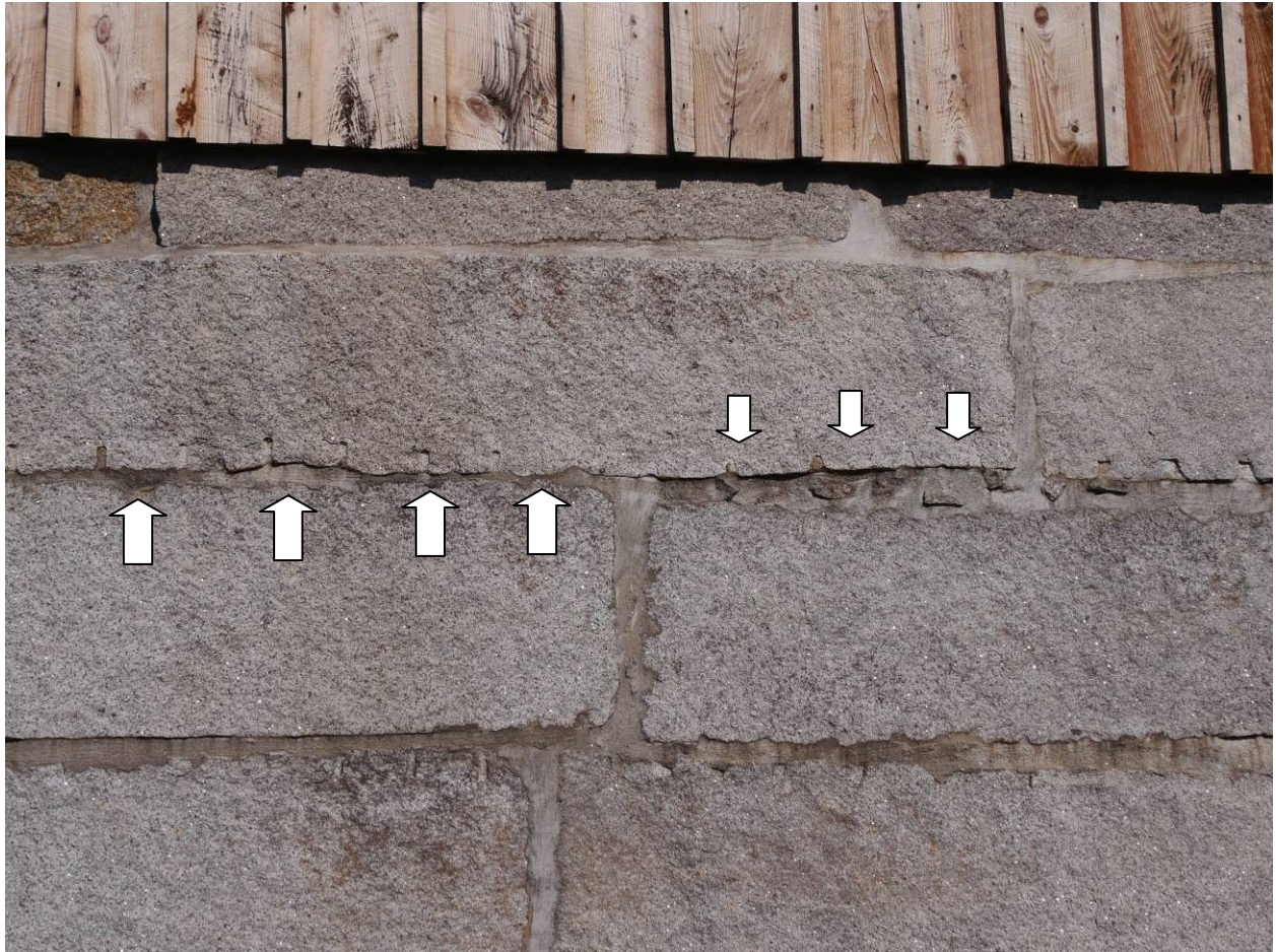
A single bar of granite was found split using both methods: Flat wedge method (down arrows) and plug & feather method (up arrows).
