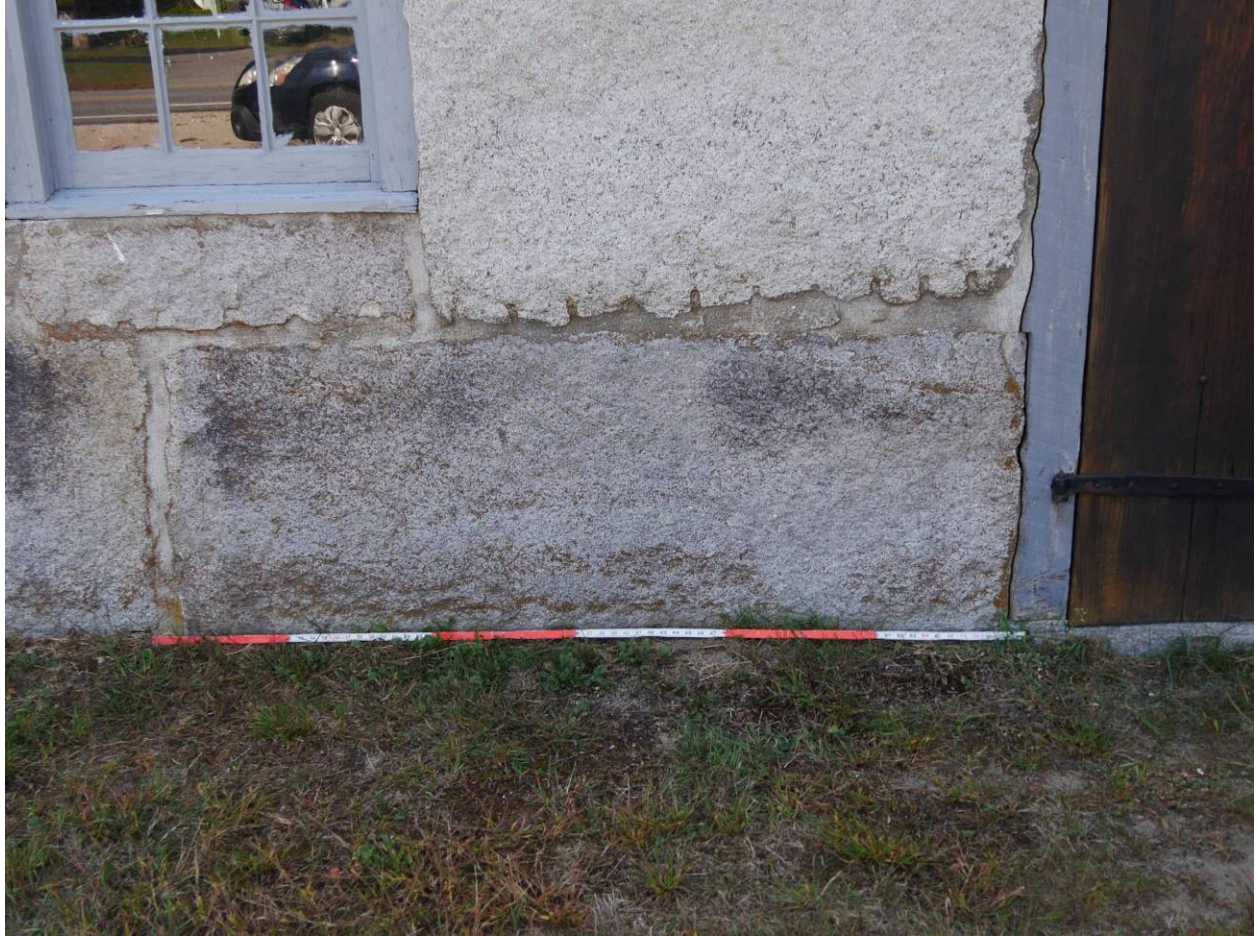
Stone block to the left of main shop entrance on the front of the building. 5 ½ x 2 x 1 ½ feet in size weighed in at around a ton
