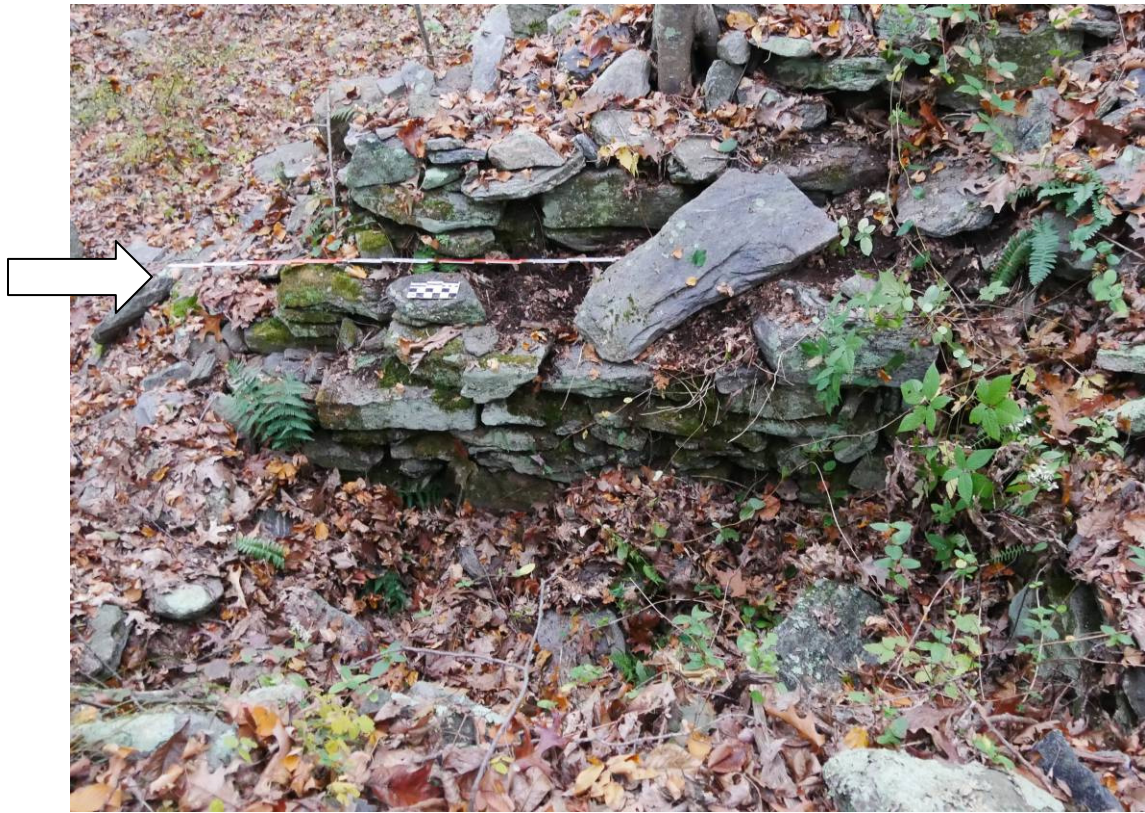
Figures 21 & 22 - The scale ruler marks a physical seam between the north side of the chimney block and the room added on the north side of the house. The shelf like stone work addition may have been part of the brick oven reportedly excavated at this location.
