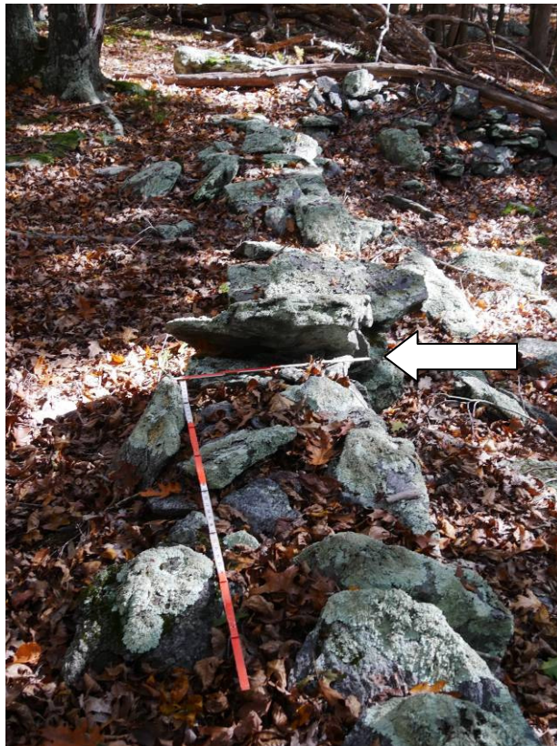
Figure 26 – The wall of the structure averages two feet wide, sufficient to support a wooden structure
