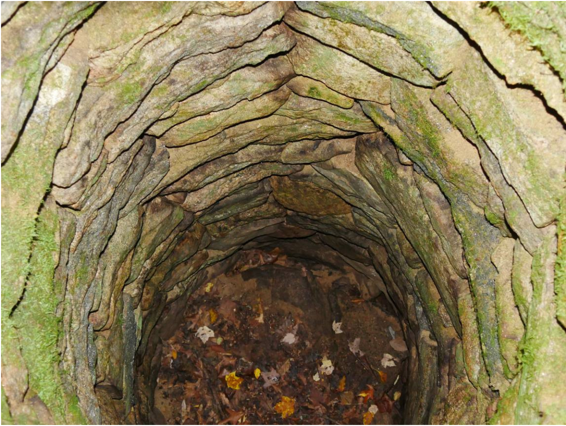
Figure 10 - Interior of well
