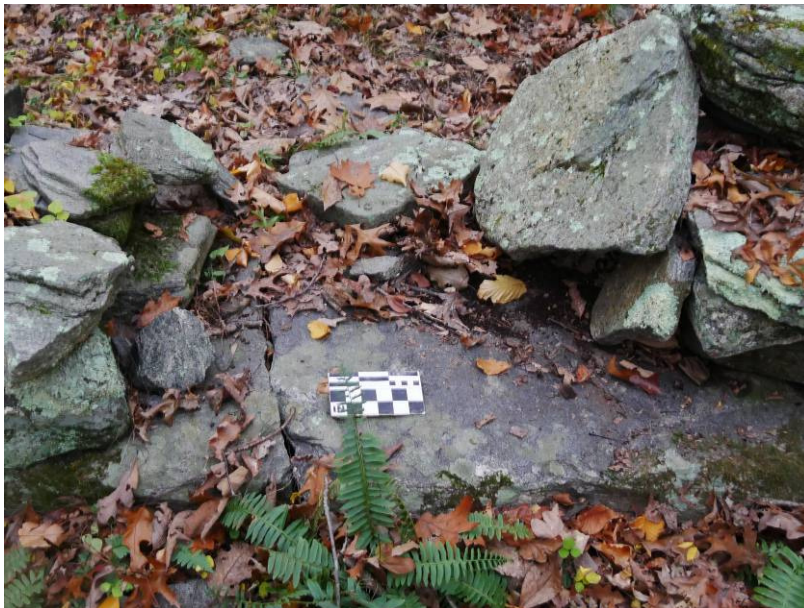
Figure 18 - Threshold stone in south wall of foundation for entry into the house
