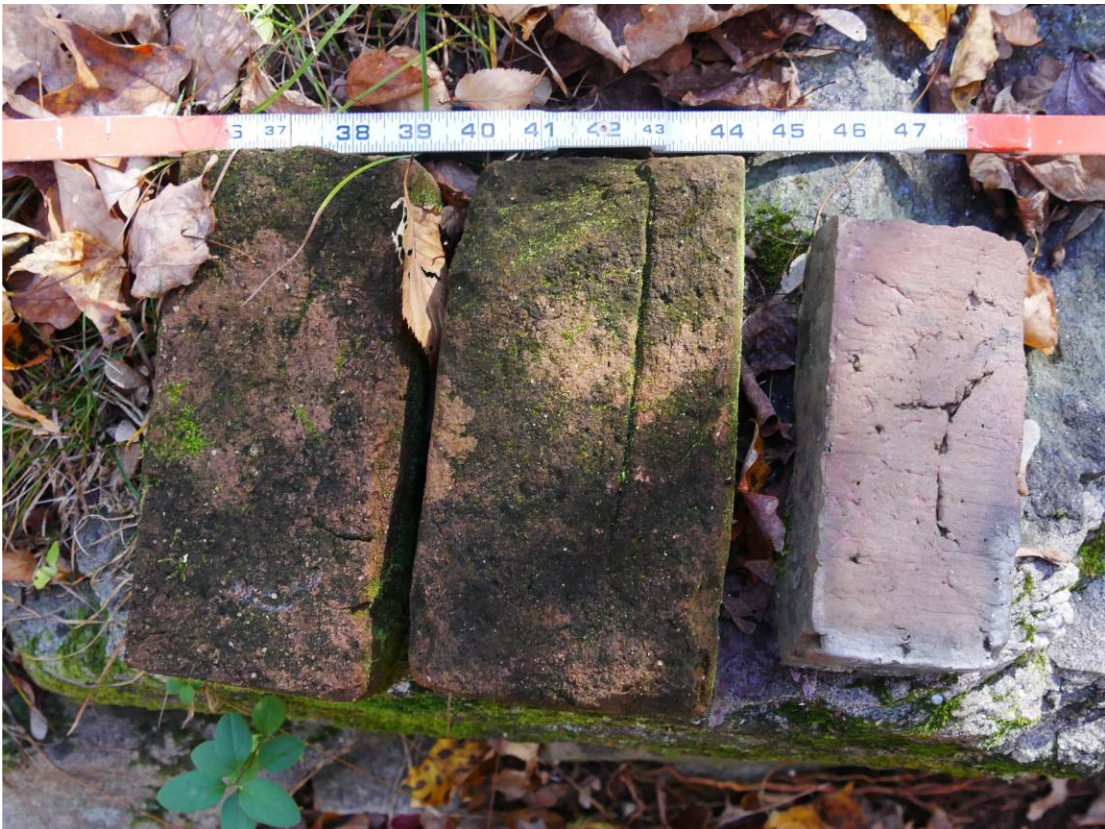
Figure 8 - Bricks placed on top of the wall of the cellar entry (top down view)
