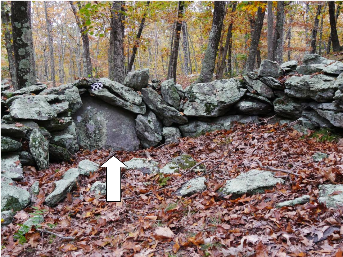
Figure 27 & 28 – Boulders embedded in wall of the structure (top) south wall (bottom) west wall
