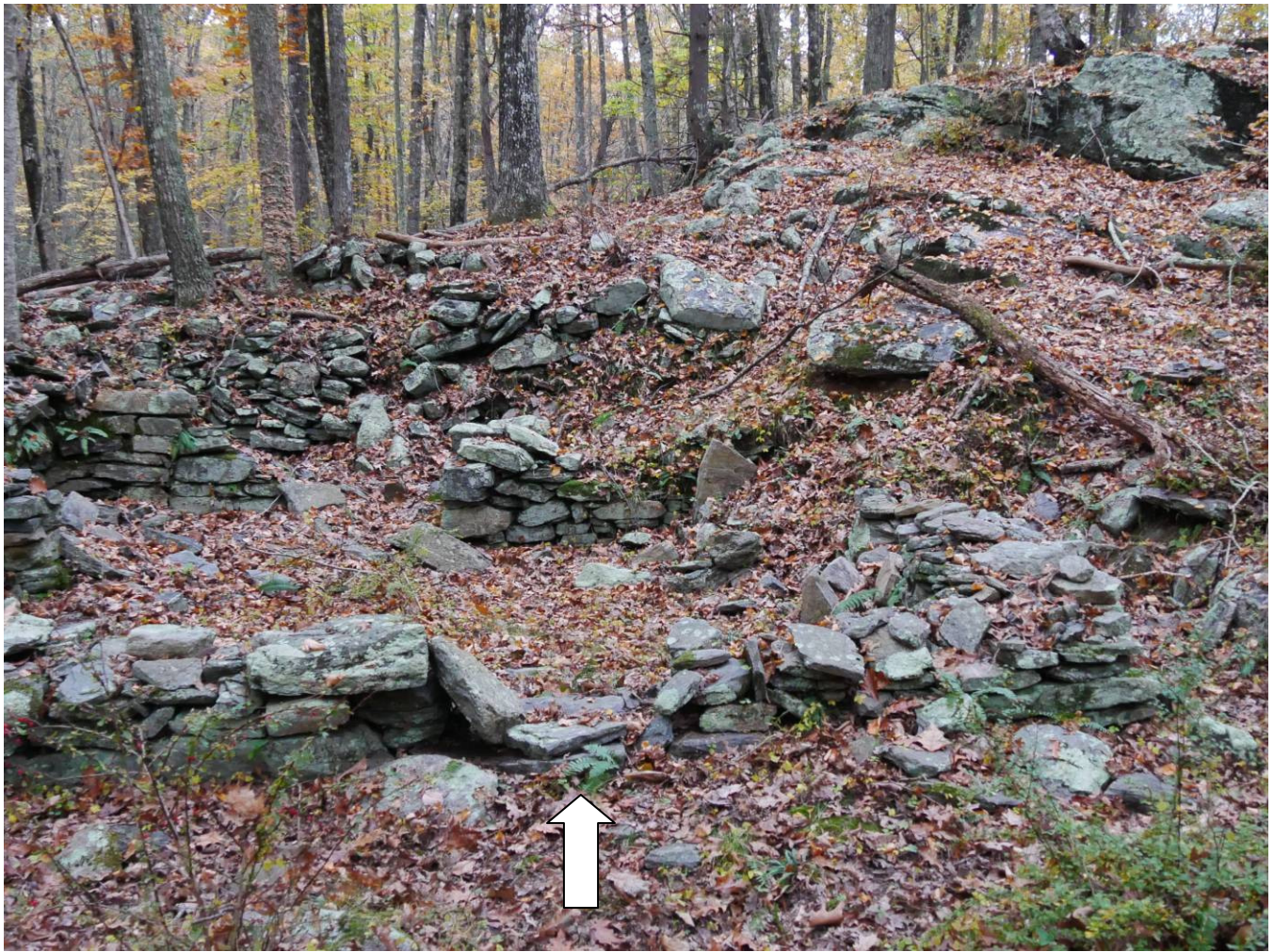
Figure 17 - View of Adams house foundation on west side of farm looking north. Arrow points to threshold stone for entry.
