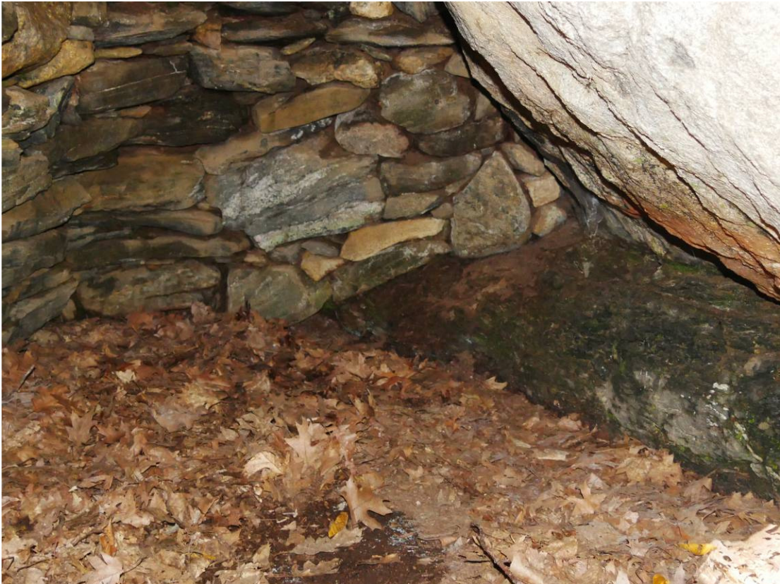
Figures 39 – Interior views of Chamber #2 with large anchor boulder
