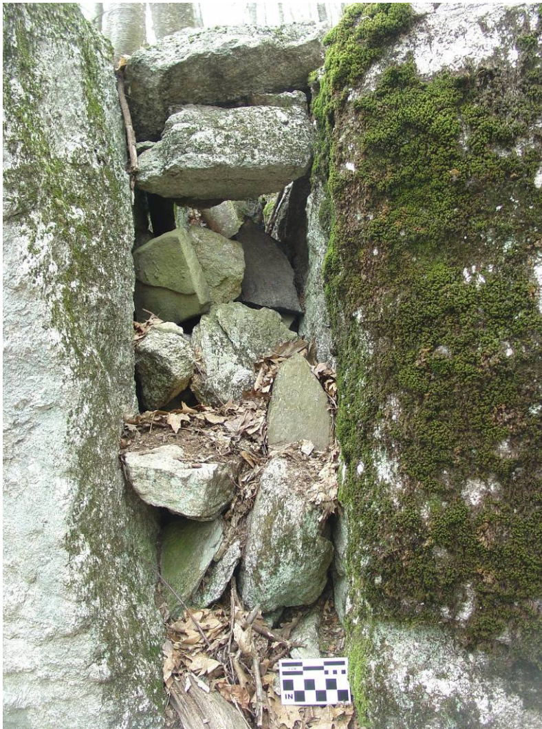
Figure 8 – Close-up view of stones placed in the split
