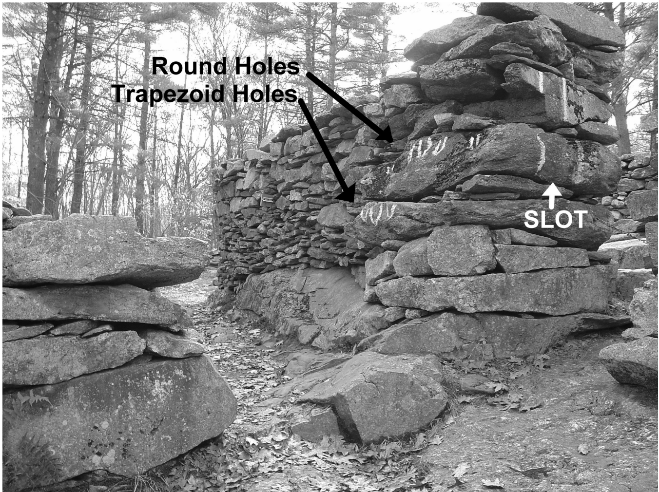
Figure 13 – The north end of the Tall Wall structure showing the abraded slot. The quarry marks from an 1860's operation to remove stone slabs from the site are visible on the east side.
