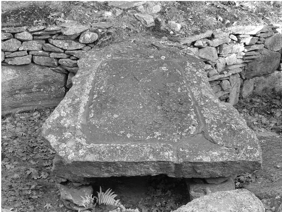
Figure 9 – The Grooved Stone rests on four stacked stone columns and the edge of the Oracle Chamber. It is in its original unaltered position.
