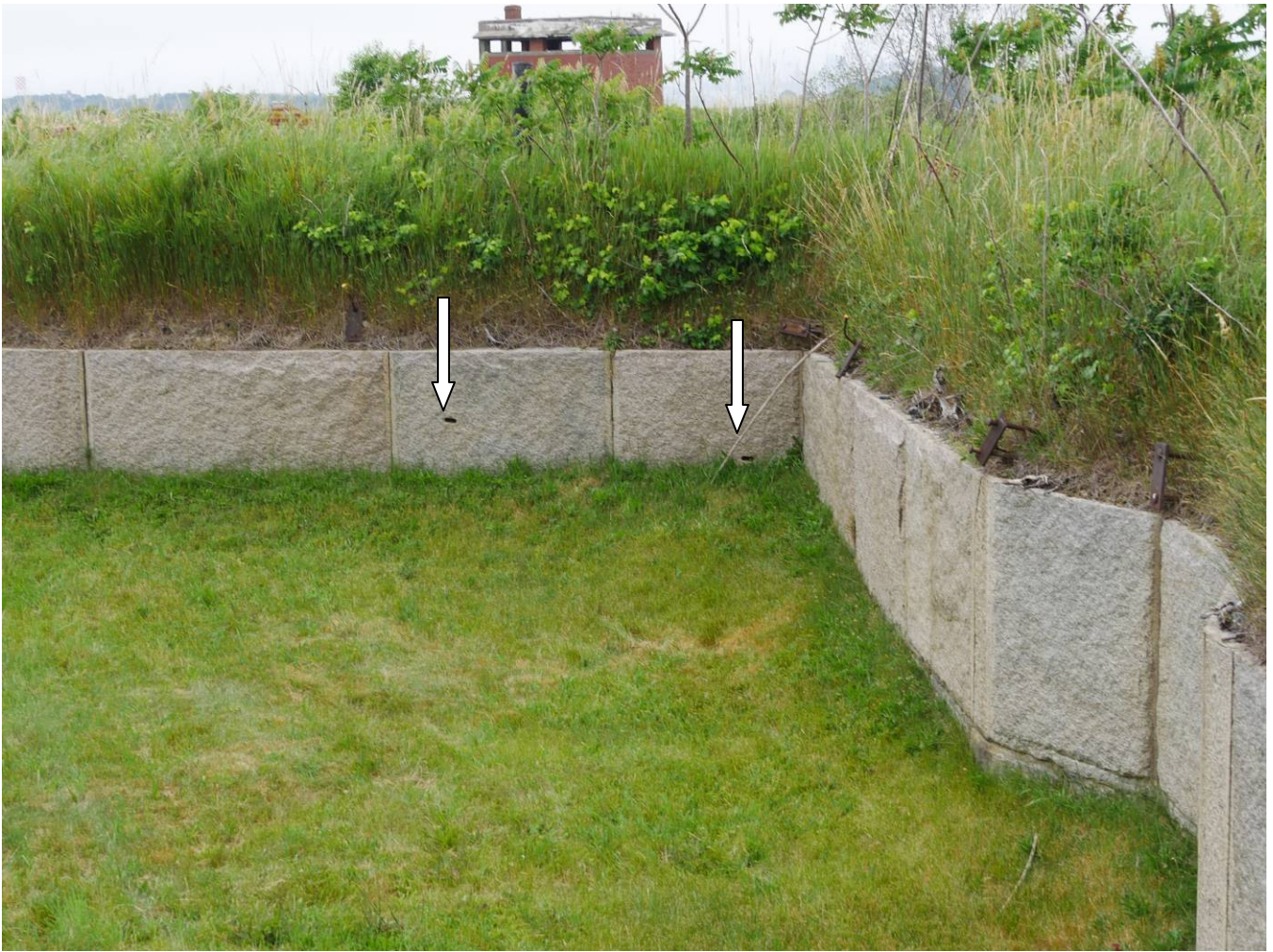
Figure 27 – Lewis holes at location No. 7 on map are also not in the center of the block either/
