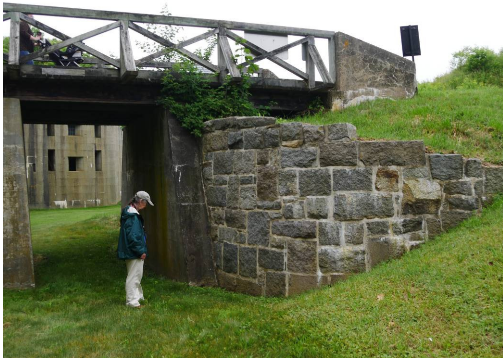
Figure 6 – The hand cut flat wedge holes were found on a single block in the sally port bridge retaining wall
