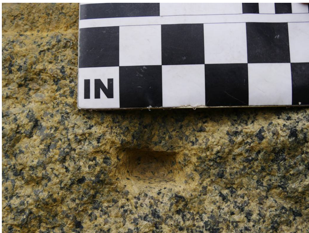
Figure 11 – A shallow flat wedge hole cut with a cape chisel and used as “dog hole” for lifting the block into place.
