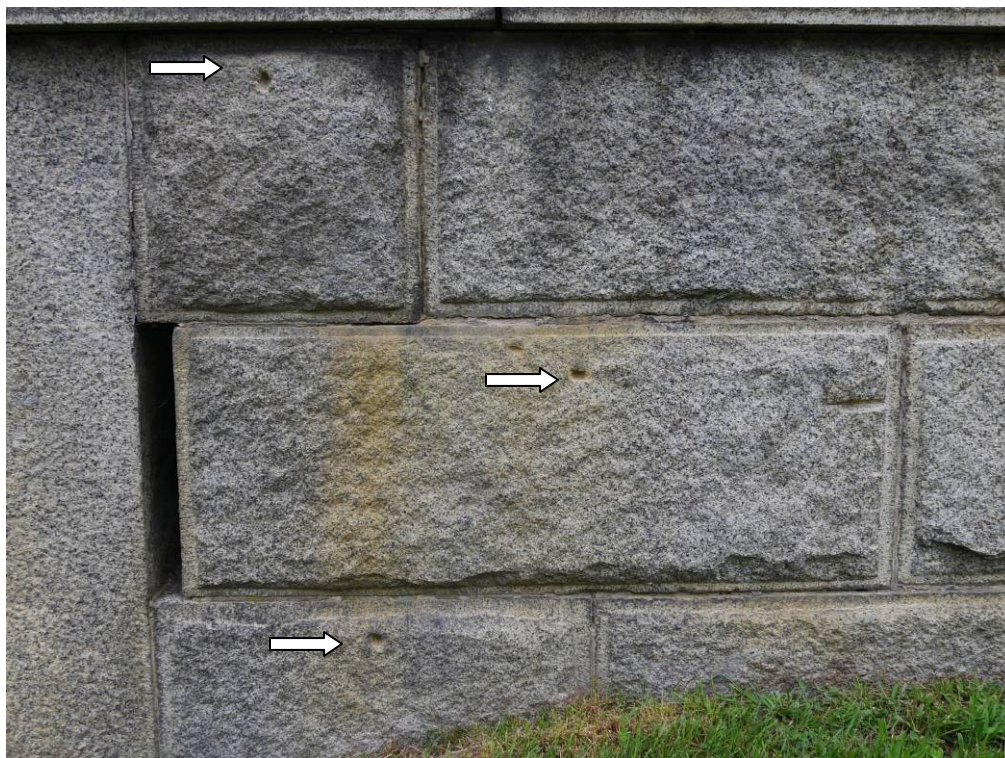
Figure 9 – Three of the blocks in this wall have dog holes near the top center of each block. Location #5 on map (Dog holes indicated by arrows)
