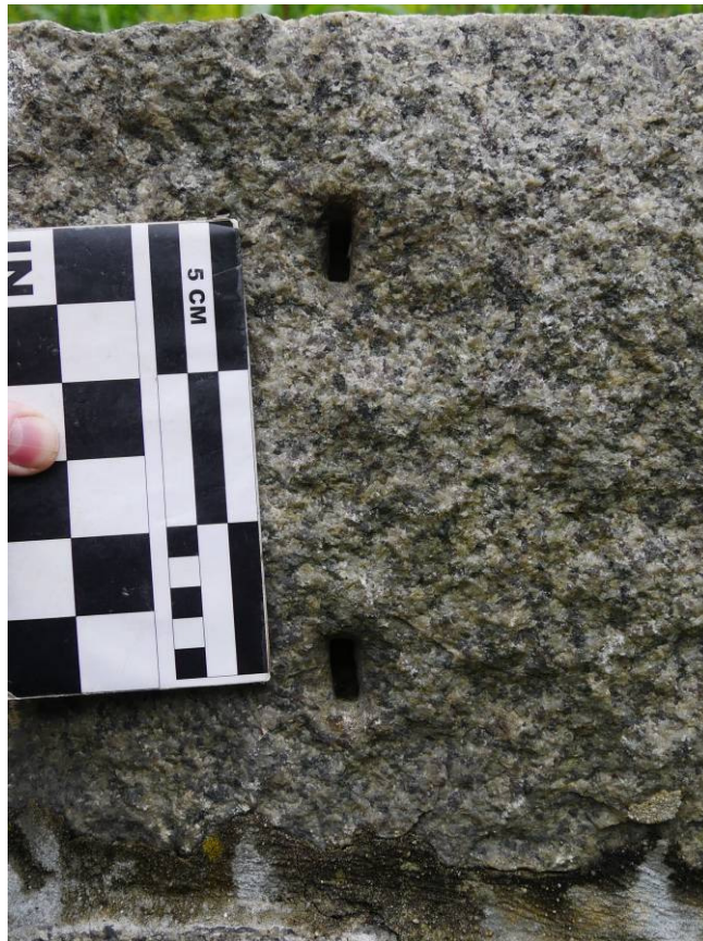
Figure 3 – Location of machine cut flat wedge holes in the retaining wall of the access road to picnic area near the demi-lune.
