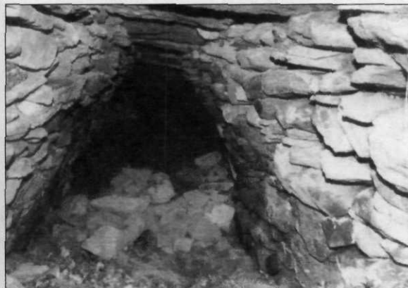
Figure 23. The Pottie Chamber has vertical to corbel walls. Charcoal found just above the roof stones produced a C-14 date of 850 BP +/- 140 years (uncorrected). Newton, NH.
