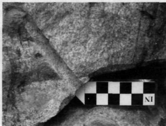
Figure 15. Some of the stones used in the barn foundation were blasted field stone. This foundation stone has a single long blast hole.
