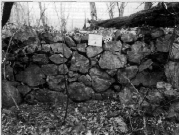
Figure 12. House foundation with flat faced walls, square corners, and box-like shape. Georgetown, MA.
