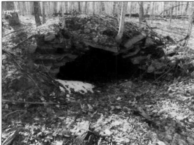
Figure 31. Exterior view of a stone chamber showing the corbelled wall to slab roof design. Hoffman Evergreen Preserve, Stonington, CT. (Photo by Ted Hendrickson, used with permission.)
