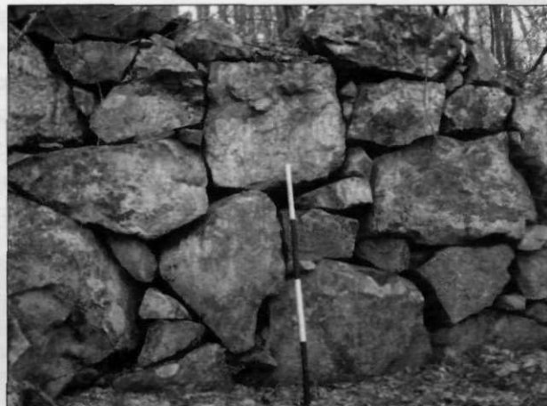
Figure 14. Barn foundation has the same characteristics as the house foundation in figs. 12 & 13. The only difference is the flat faced stones are larger. Georgetown, MA.
