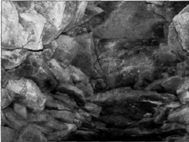
Figure 6. Fully corbelled chamber (dome roof), Rocky Brook Stone Chamber, Thompson, CT.
