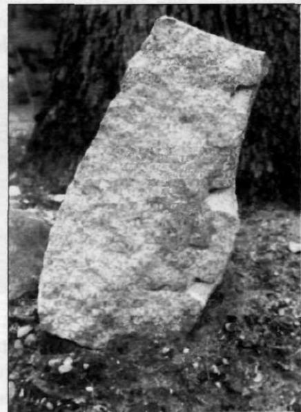
Figure 21. Trapezoid shaped tool marks from the flat wedge method of splitting stone.
