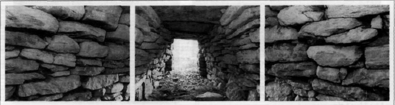
Figure 17. This root cellar has a rectangular tunnel like room with long parallel vertical walls that transition to corbelled near the top. Montville, CT (Photo courtesy of Ted Hendrickson).
