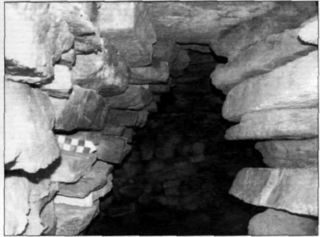
Figure 7. Corbel to stone slab roof construction, stone chamber, Webster, MA.
