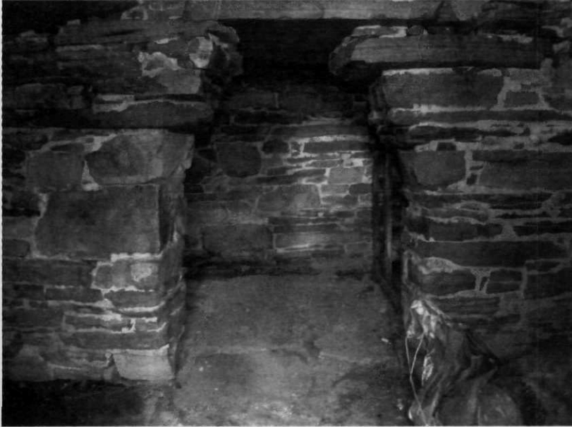
Figure 9. This root cellar is divided into four rooms by two thick stone masonry walls which double as columns to support the stone roof. Three layers of corbelling are evident at the top of the walls. Spicer Hill Root Cellar, Ledyard, CT.
