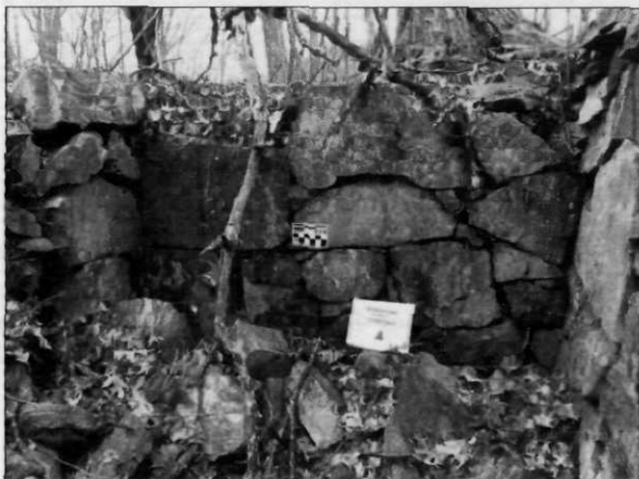
Figure 13. Another wall of the same house foundation showing the common type of flat faced stones used.
